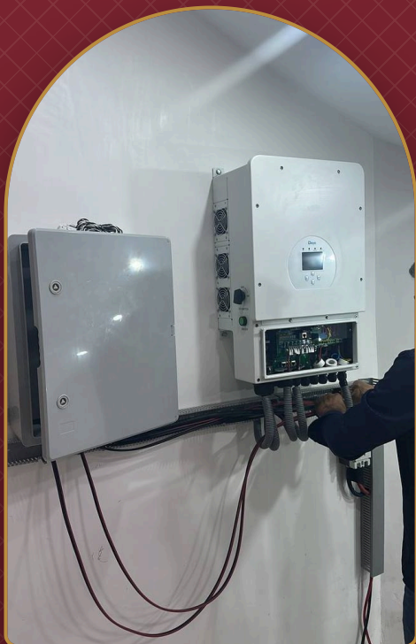
AC / DC TERMINATION WORK
