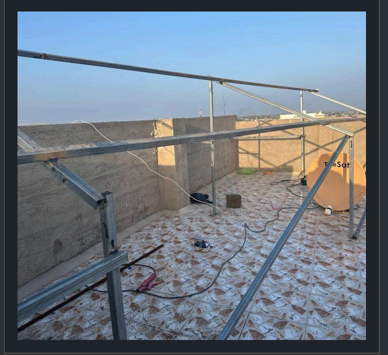
GALVANISED ROOF FRAME — PREPARED FOR PANELS
